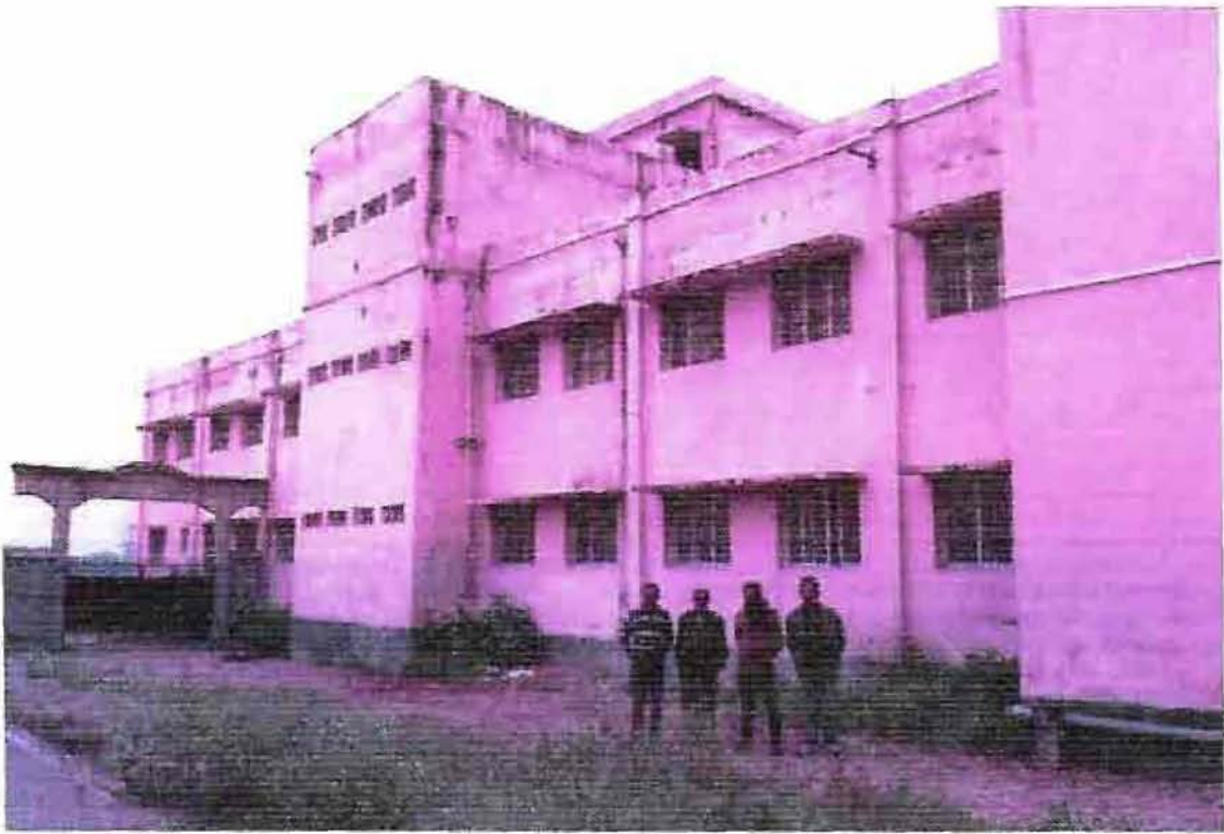
Rear view of the building
